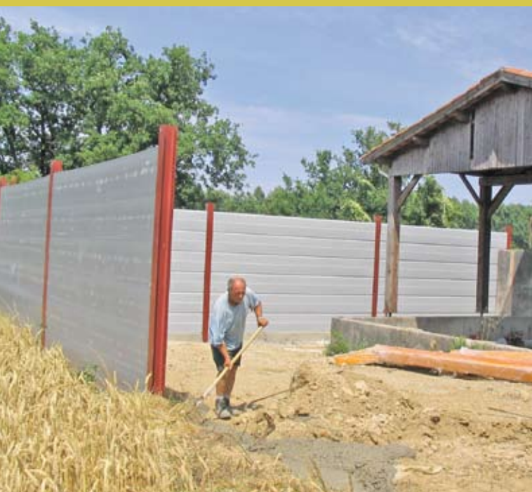
Vandpumpestation, St-Sulpice (F)
